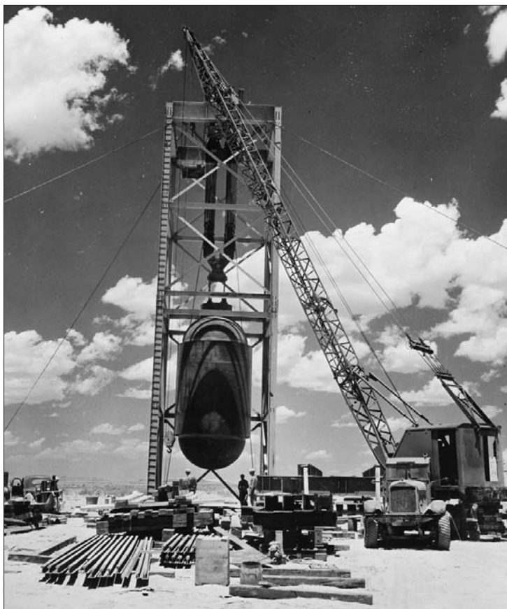
First atomic bomb being readied on a 100-foot-high tower at the Trinity Site.
