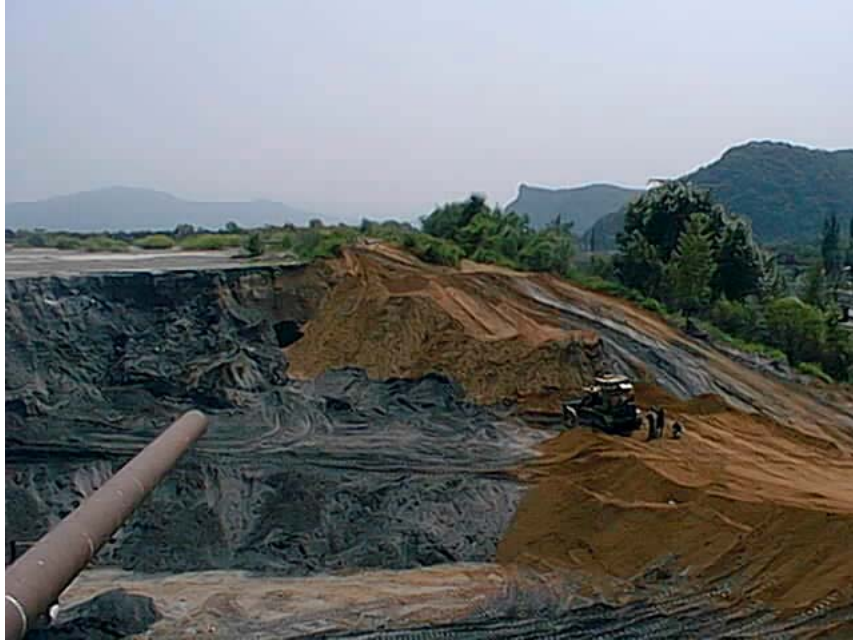
4 of 7 - View of breach zone from within the ring dike dam
