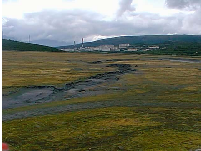
6 of 7- View of full coal ash disposal dam - a ring dike - at primary power plant at Magadan City located in flood plain of Magadan River
