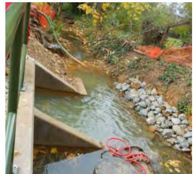
9 - Treated water enters stream where contaminated water used to flow
