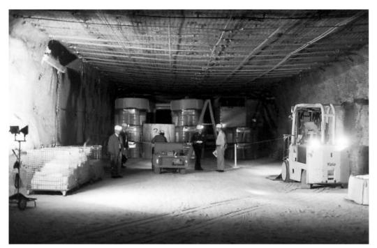
Picture 2. The north end of Room 7, Panel 1 and S1600 drift on March 4, 1998. The roof support consists of roof-bolts, wire and cables. Behind the drum stacks is the ventilation barrier with two louvered exhaust openings separated by a large roll-up door.
