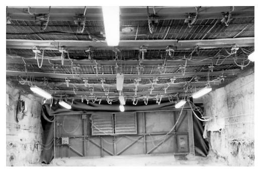
Picture 1. The north end of Room 1, Panel 1 on March 4, 1998. The roof has a specially designed support system and roof-bolt sensors. The ventilation barrier has two adjacent louvered exhaust openings.
