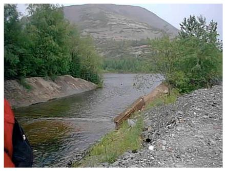
View of Inlet to Diversion Channel without Pillars to Prevent Intrusion of Ice into Diversion System
