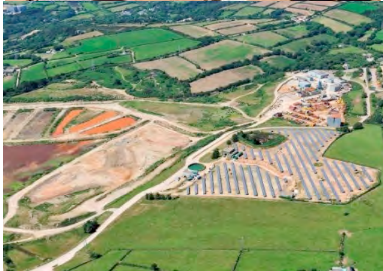
Cornwall, England – 1.4 MW photovoltaic system at former tin mine – at:
