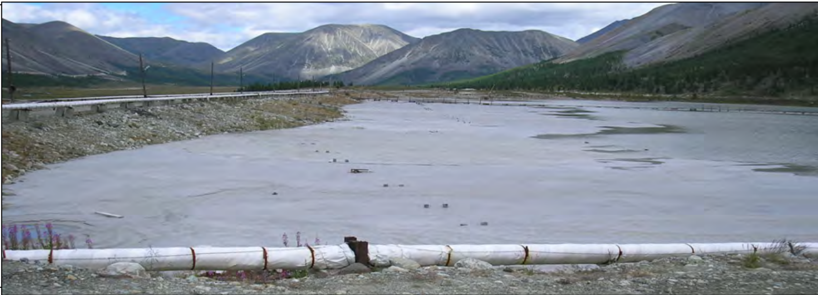
Samarta Tailings Dam, Buryatia - Example of (1) tailings beach established to keep liquids from saturating dam, (5) use of multiple tailings discharge points to establish thin layers of tailings to reduce infiltration potential and (6) tailings liquid recycle to reduce volume of liquids behind dam.
